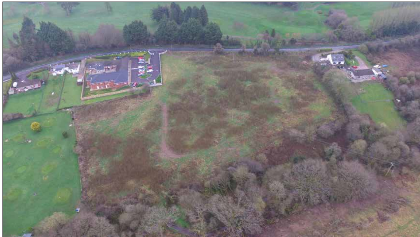
Plate 11.3 Aerial view of Field 2, looking north
